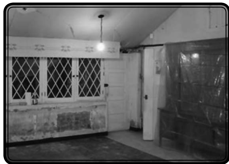
The kitchen undergoing repairs and repainting—Photo: Davey Willans
