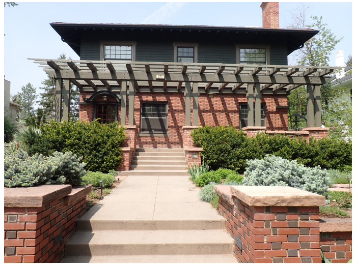
Fig. 5 The Craftsman house at 171 Franklin. Dramatic shadows cast are by the porch beams. The Flemish brick work of the walls is seen to advantage in the column in the foreground.
