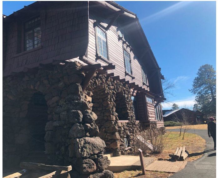
Parts of the Riordan Mansion: in the foreground, the West house, constructed of local ponderosa pine – 2nd story: shingles, in the shade, planks, in the sun; 1st story, applied slabs (right), eaves protruding, local basalt rock. In the distance, far right, is the East house.
