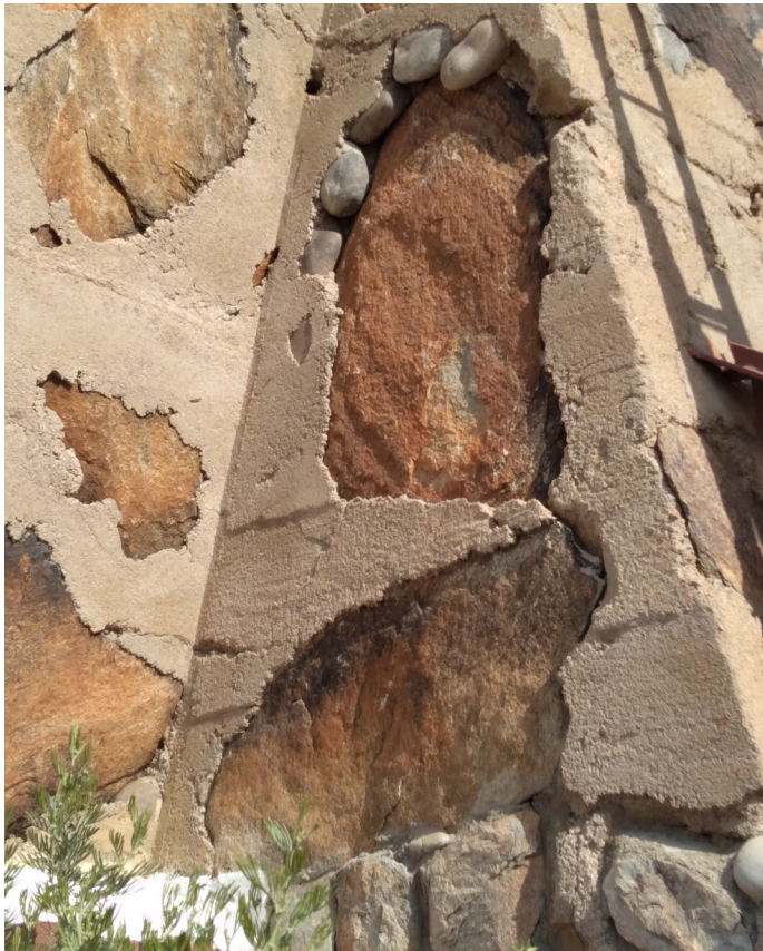
Fig. 7. Construction of Taliesin West walls: desert rocks and sand, held together by cement.
