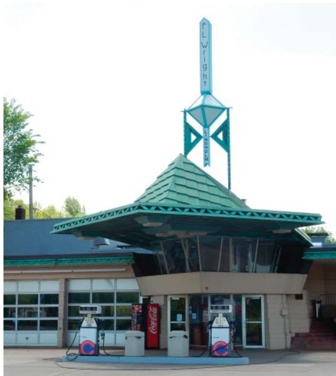
The only FLLW gas station, the Lindholm Service Station in Cloquet, MN. An octahedron decorates the sign. The pylon rises from the copper canopy, from which the gas hoses were to hang.
