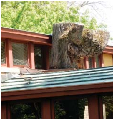
Tree growing through the porch of the Isabel Roberts House, 1908. The Roberts House was not a part of the tour, but was pointed out, as next door to the Drummond house and done by FLLW. It nicely illustrates the Arts & Crafts philosophy of merging with nature – though here nature has gotten out of hand and threatens the structure of the house.
