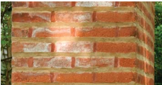
One of the ways Wright provided horizontal emphasis was to suppress the vertical lines and expand the horizontal lines of mortar between bricks.
