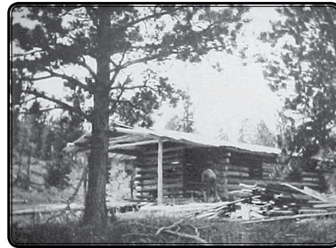
A guest cabin being built on Ten Sleep Ranch
