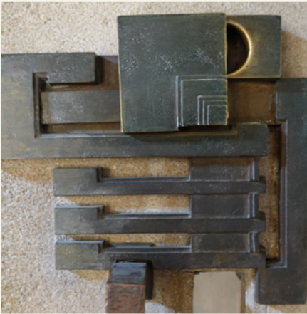
Fig. 1. Front door lock. The keyhole, at the top, can be hidden by the brass fixture, here half-way drawn.
