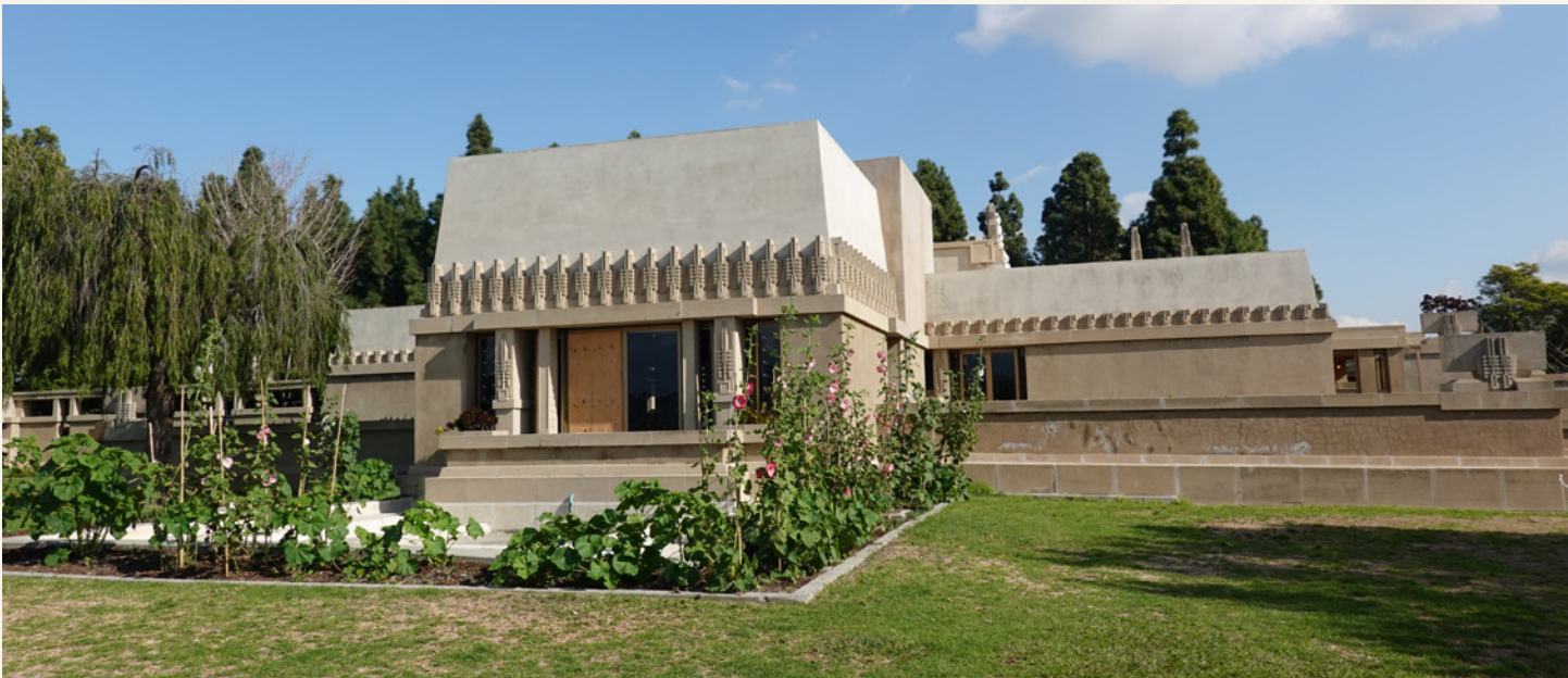
Fig. 2. Hollyhock House in Hollywood, from the West. Note the sloping walls, and cast-concrete Mayan-like ornamentation.
