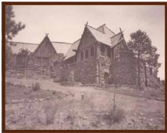
Southwest elevation showing covered porch and dining room.
