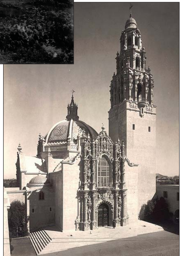
California Bell Tower
